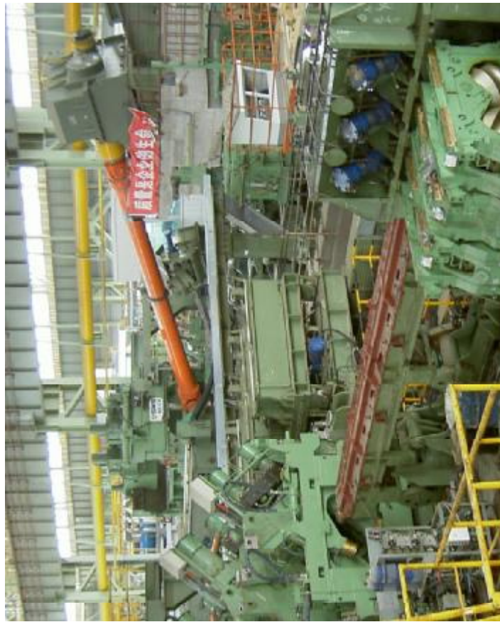
攀成阳无缝钢管机组 Pangang Group Chengdu Steel & Vanadium Co.,Ltd.Seamless Steel Pipe Unit
